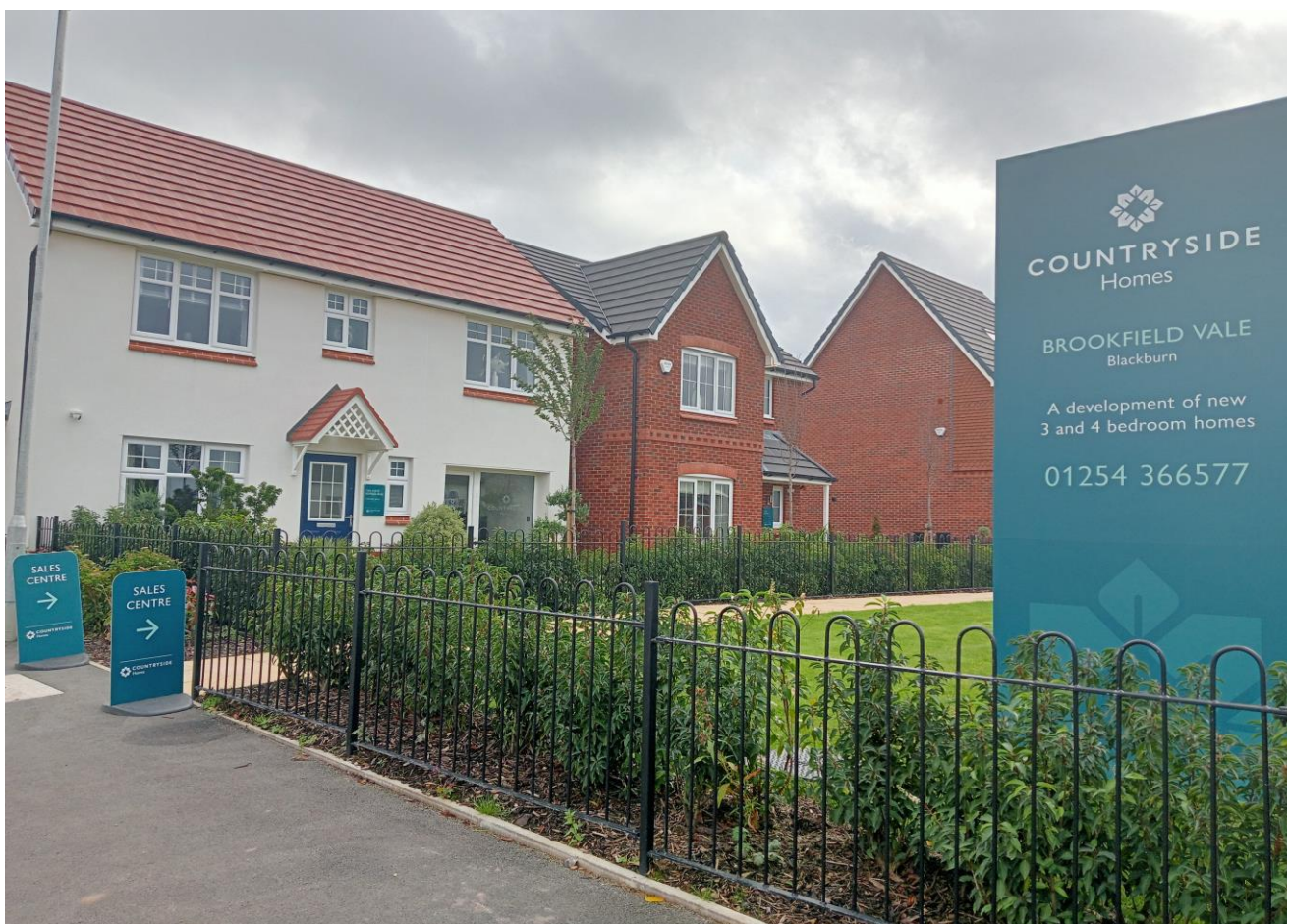
S106 contributions have been secured from the Countryside Homes development on Roman Road, Blackburn
